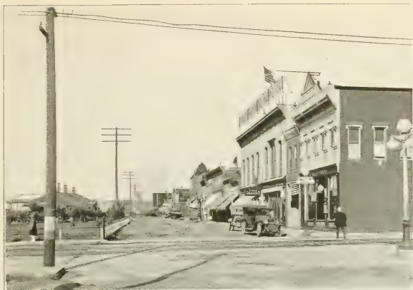
SOUTH FRONT STREET, ROCK SPRINGS
