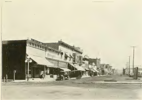
NORTH FRONT STREET, ROCK SPRINGS
