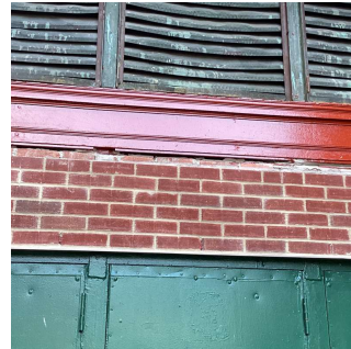
Facade A - Near HC Entrance
