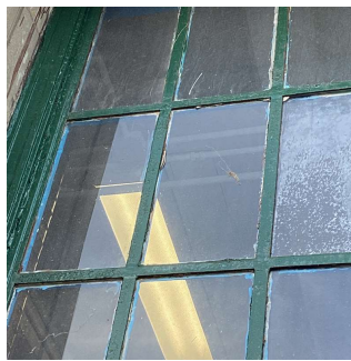
Facade A - East Entrance No violations recorded.
