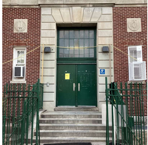
Facade A - 17th Street
