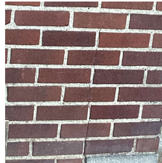
Facade D - North Entrance
