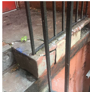
Facade C - Exit 2
