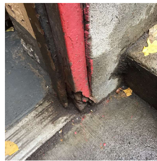
Facade M - Boiler Room Exit at AW5 35636275K
