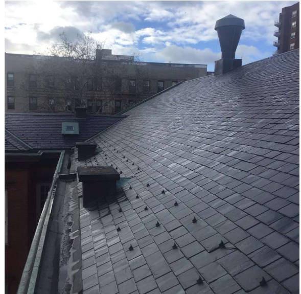
Roof 1 - South View
