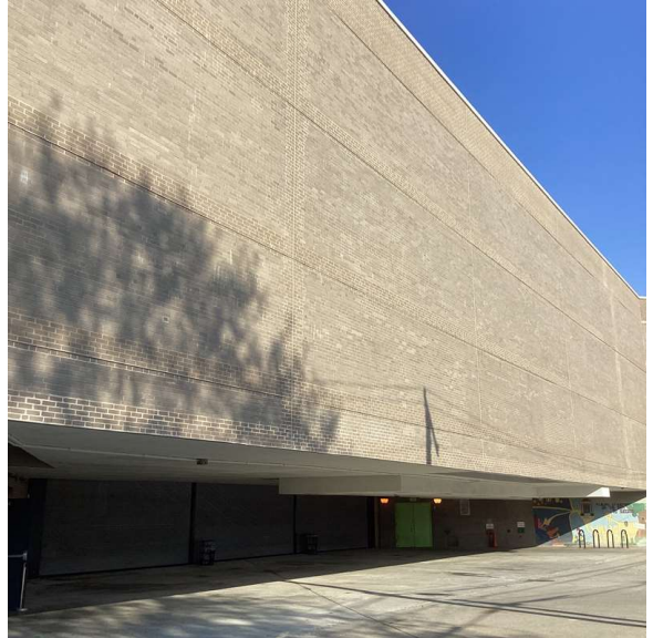
Nameoke Street - Northwest view
