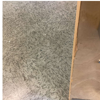
Entrance No violations recorded.
