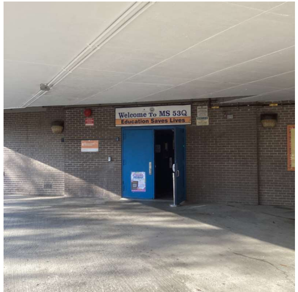
Facade A - Nameoke Street
