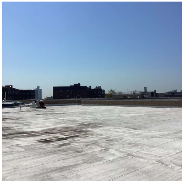
Roof 1 - South view
