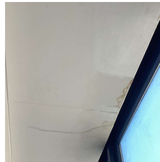
Facade K - Skylight at Corridor near Room 381, also Skylight Room 301
