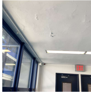
Near Room 170 No violations recorded.
