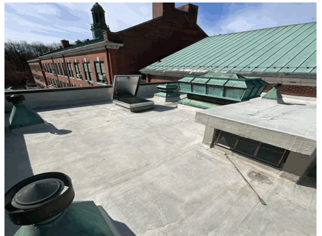
Roof 10 - South View
