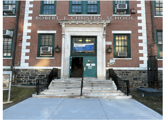
Facade A - Riverdale Avenue
