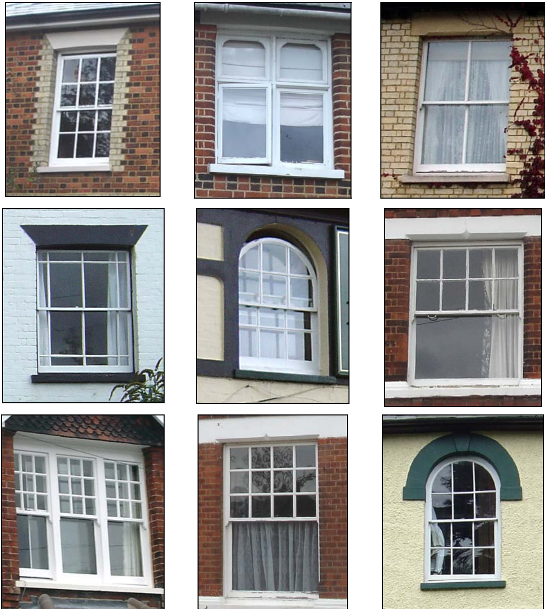
Figure 26. Some examples of the original 19 th and early 20 th century timber window styles within the Orchard Road Conservation Area
