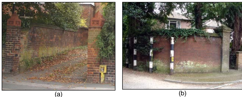
Figure 25. Red brick walls and associated red brick gate piers with decorative terracotta caps on Julian's Road (a), curved red brick wall to north of 5 Orchard Road (b)
