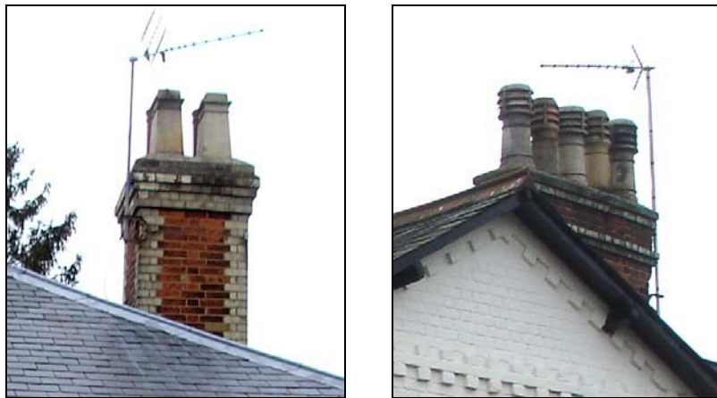
Figure 24. Chimney stacks and chimney pots within the Orchard Road Conservation Area
